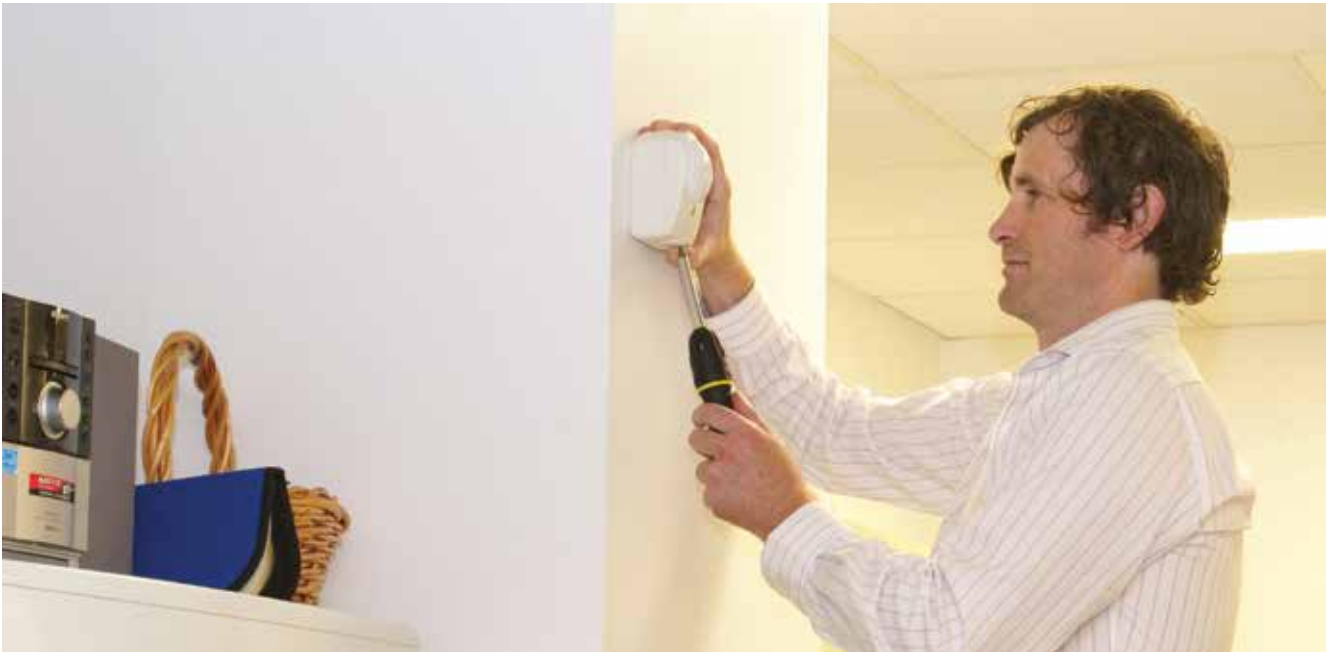
Installing Inactivity Sensors
